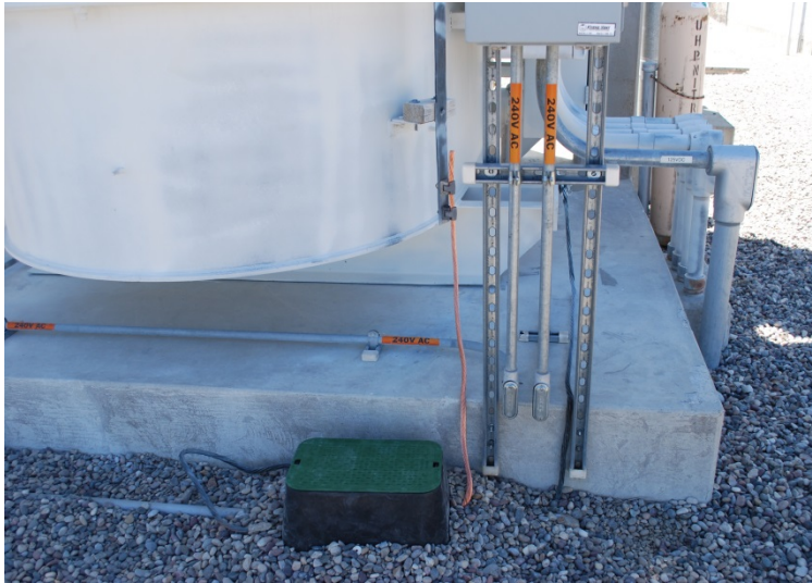
Figure 1. INL Typical INL Transformer - GMD Ground Current Measurement.
